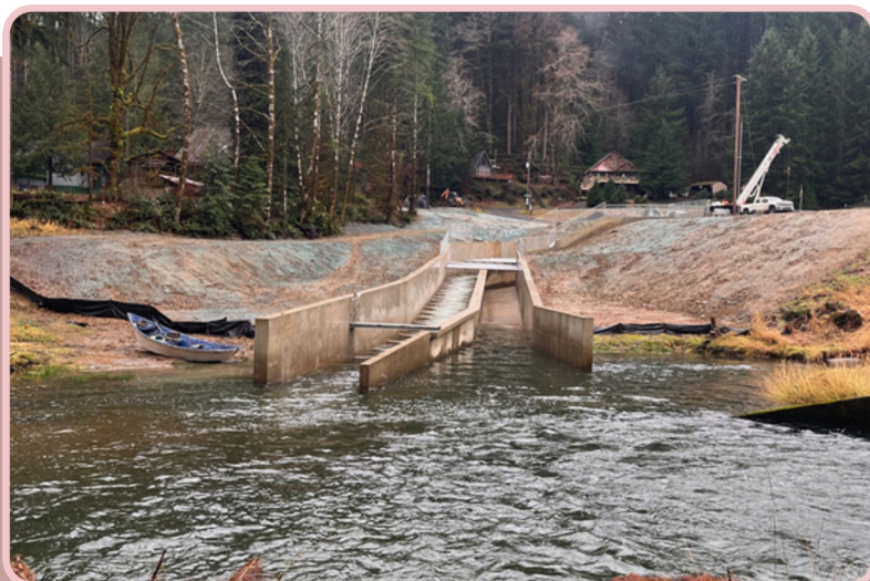
New fish ladder completed at Fishhawk Lake in 2023
