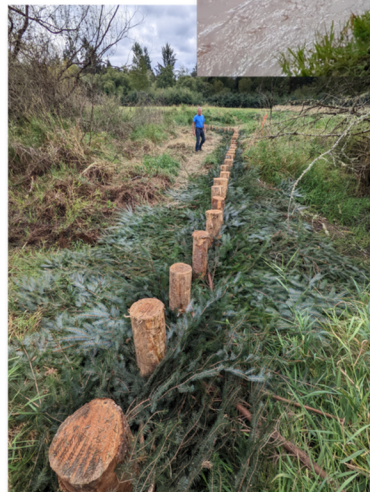
Newly installed Beaver Dam Analogue
